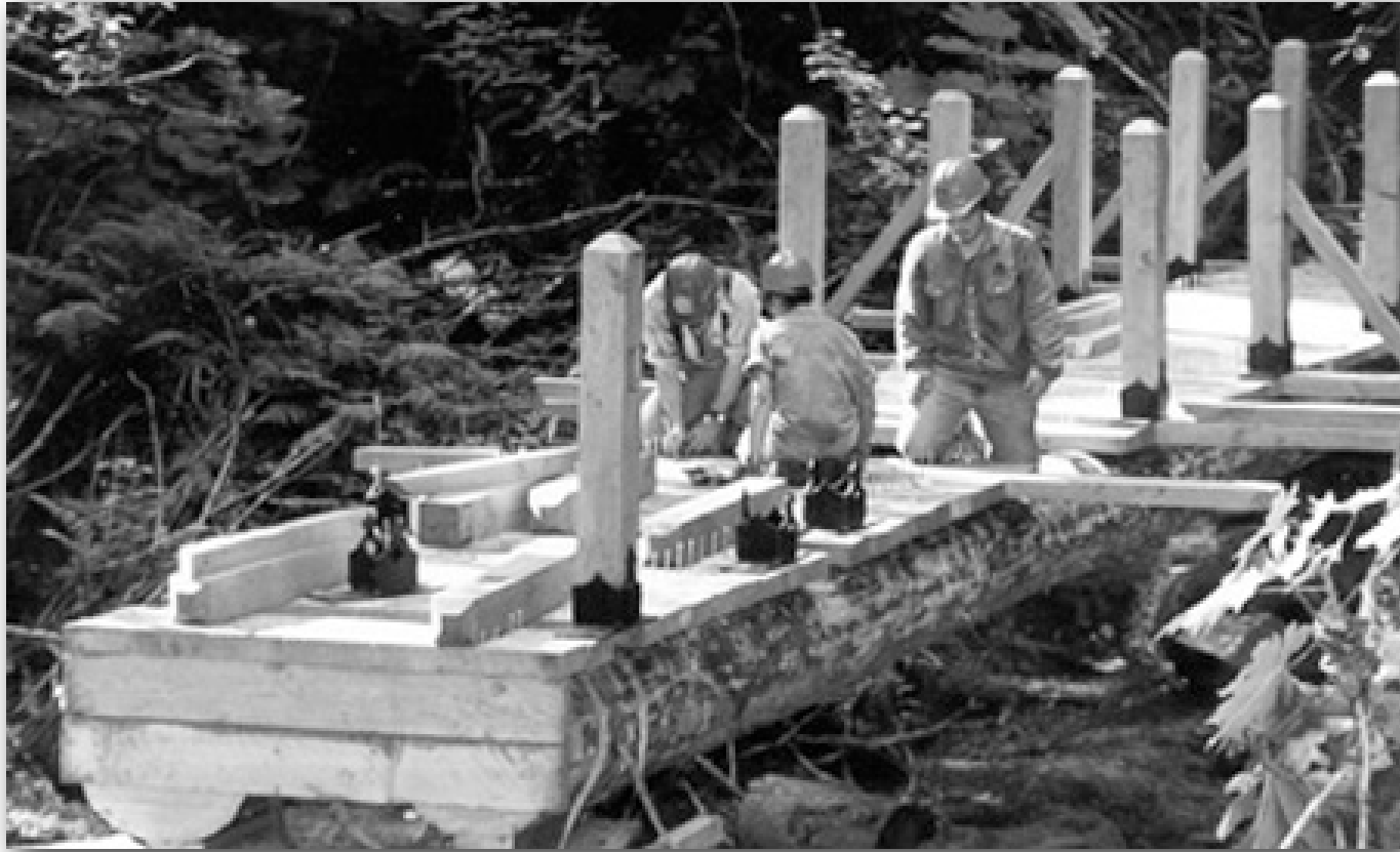
Northwest youth corps building a bridge (NWYC, 2000)
